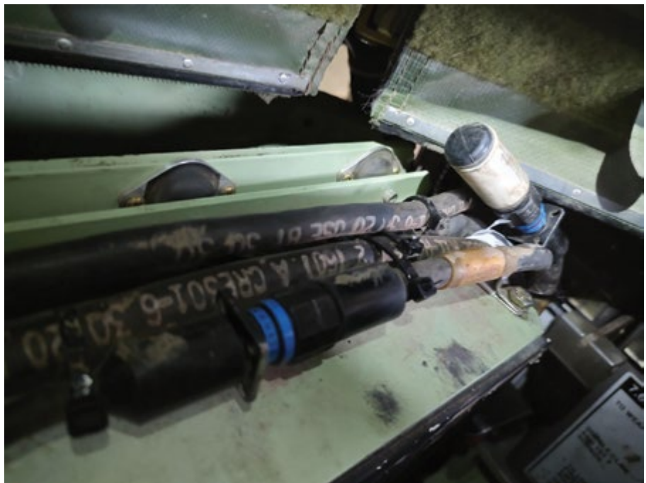
Figure 5. Image of CAN bus cables without bracket installed. (Image by SFC Donald Fadel)
